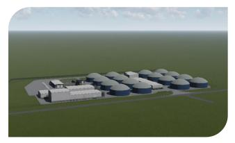
By removing nearly half of the digestate volume as clean water, the facility helps reduce the number of trucks moving digestate and minimizes the volume of material participating farms have to lagoon store and then land apply each year. Since the farms receive back more concentrated liquid digestate, they save money on land application, can use the liquid fertilizer in a more targeted fashion
